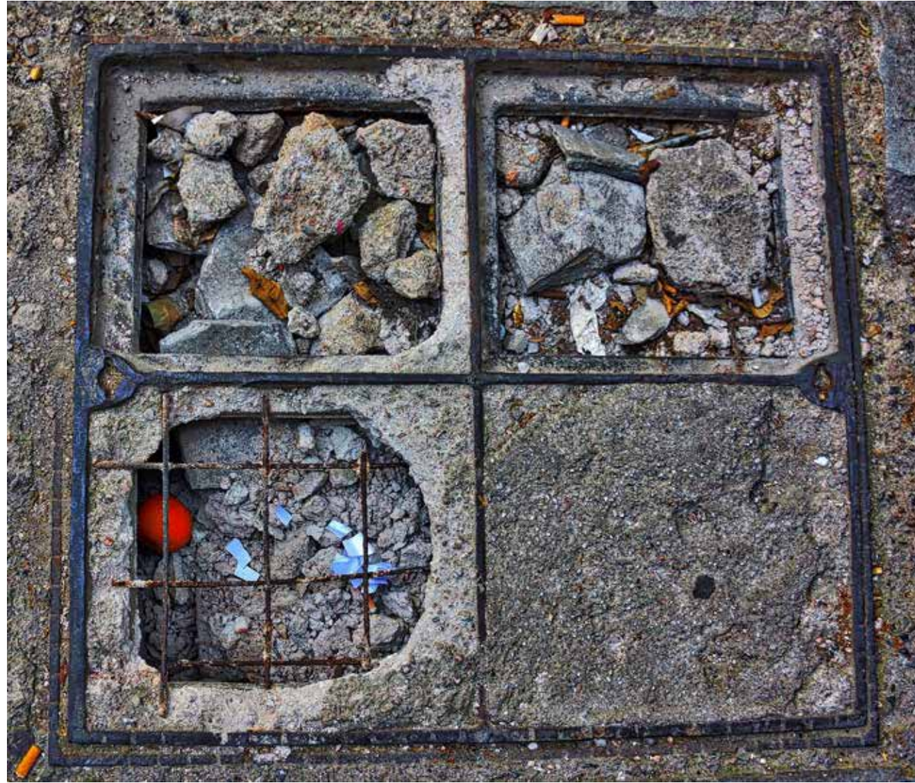
Sidewalk Grate, Athens, 2019
